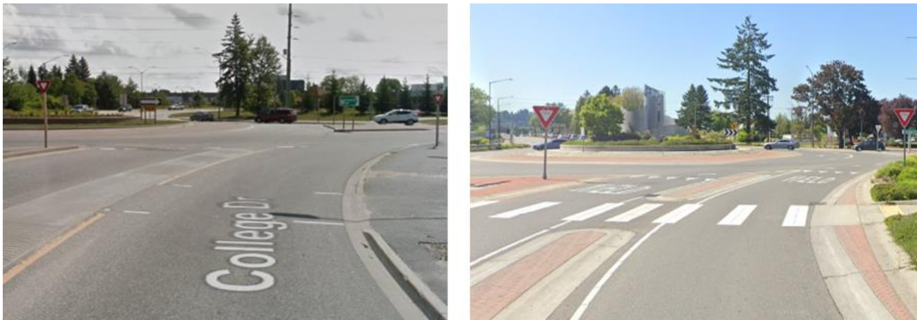
Figure 8: Example Lane Dividers using Flush Concrete with Rumble Strips (left) and Semi-Mountable Curb (right), Source: Google Street View
