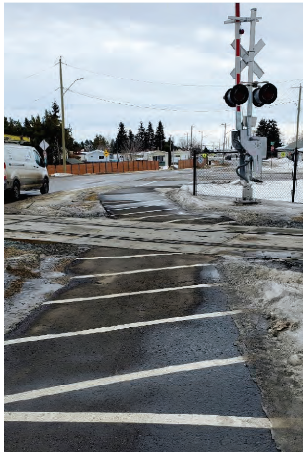
Photo 1D - Womacks Road - Pedestrian Crossing Paint Markings
