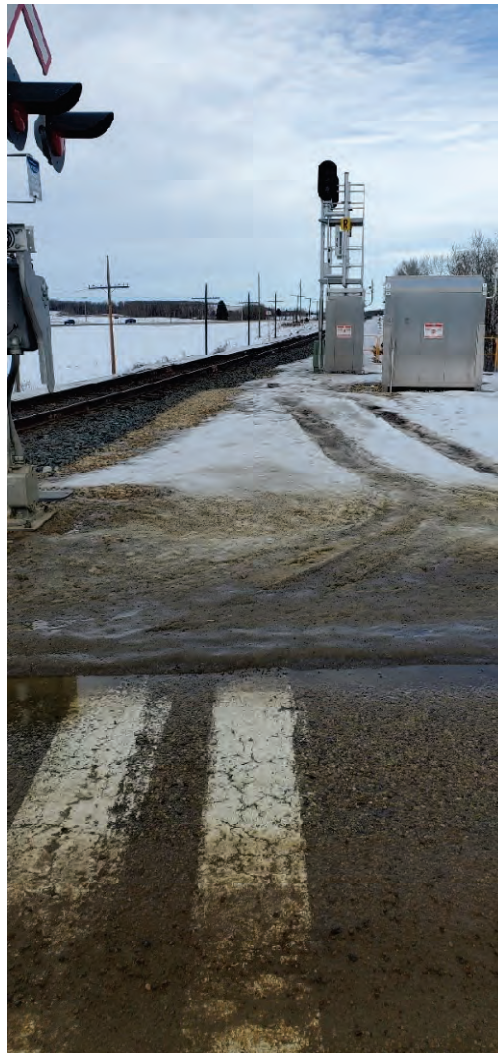
Photo 4D - Township Road 400 - Westbound Stop Bar and Obstructed Sightline North
